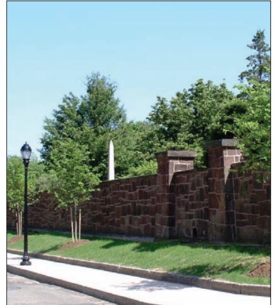
Above: View of Elm Trees on Lock Street
